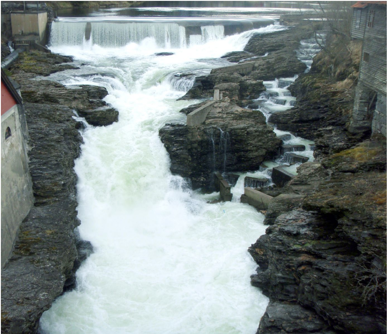
One of the “golden products” of CEDREN - environmental design of salmon rivers – was applied to Palmfossen in Vosso River to ensure increased power production and improved conditions for salmon. Photo: Hans-Petter Fjeldstad
