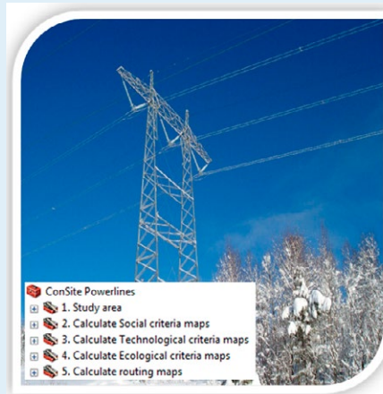
The decision analysis tool ConSite combines geographical and spatial data with stakeholder dialogue. Photo: Frank Hanssen
